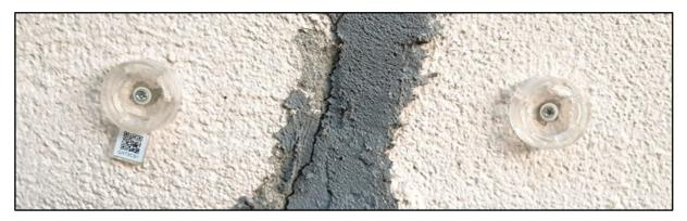
• **By gluing:** It is also possible to fix by gluing with fast-curing epoxy adhesive.
